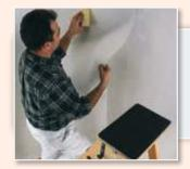
Fiberglass wall coverings with a self-adhesive layer. No need for glue nor water activation machine.
